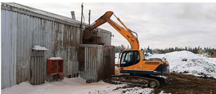
Uploading of drilling sludge to TDP for processing
